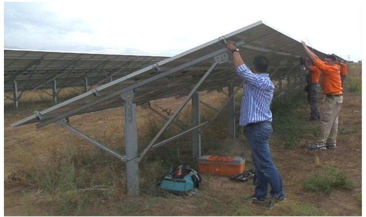
*The structure is well balanced, so a small crew of 4-5 persons can easily adjust the inclination of every stand.*
