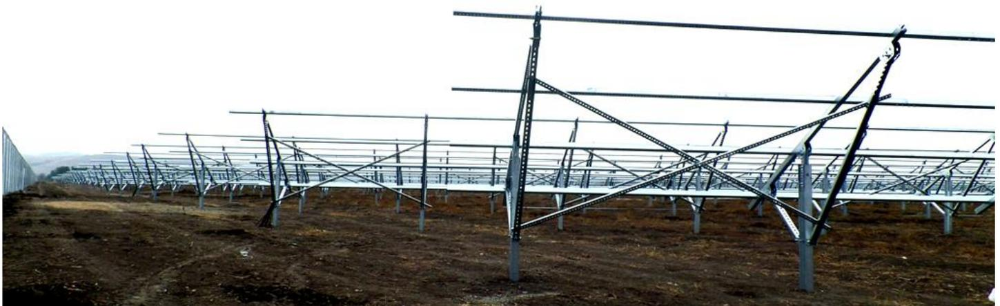
*The assembly method, with driven piles, mounting rails and components, is very flexible and gives to the constructors the ability to work fast and to encounter any problem or obstacle.*
